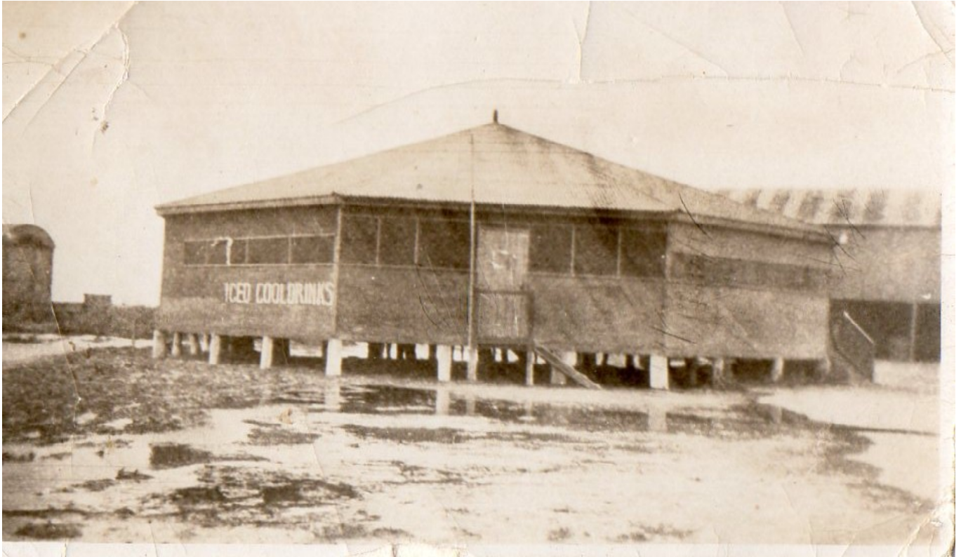
Above: The Palais after it had been raised onto pilings. Note existing railway shed and old sheds on the left.
